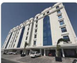
Rasiyat Al-Manar Project Jeddah, Saudi Arabia | Apartment
